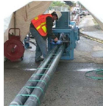
Figure 3-16. PolyFold™ Banding
