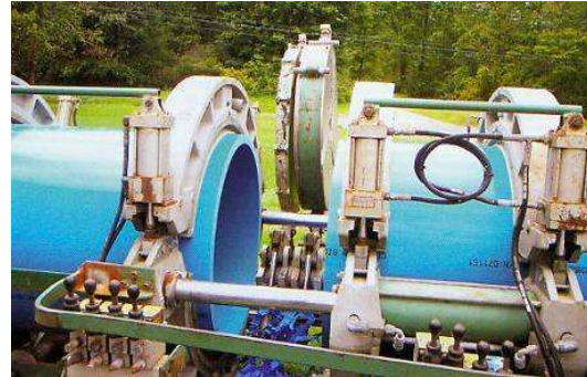
Figure 3-22. Fusion of PVC Joint
